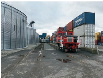
Grain railed in by train is stored in Columbia’s grain storage silos
